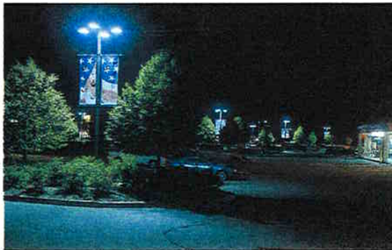
Illuminated by metal halide lamps, the reds, whites, blues, and greens in this parking lot retain their distinction and contrast. (PHOTO: GARY CLAYTON HALL)
