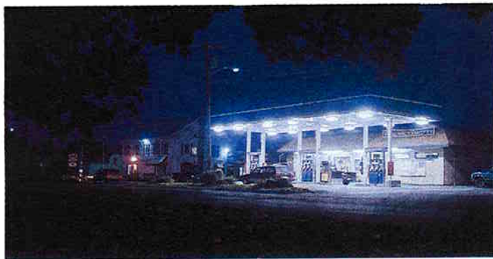
The bright light of this gas station canopy detracts from neighboring historic buildings and casts them in shadow. (PHOTO: GARY CLAYTON HALL)
