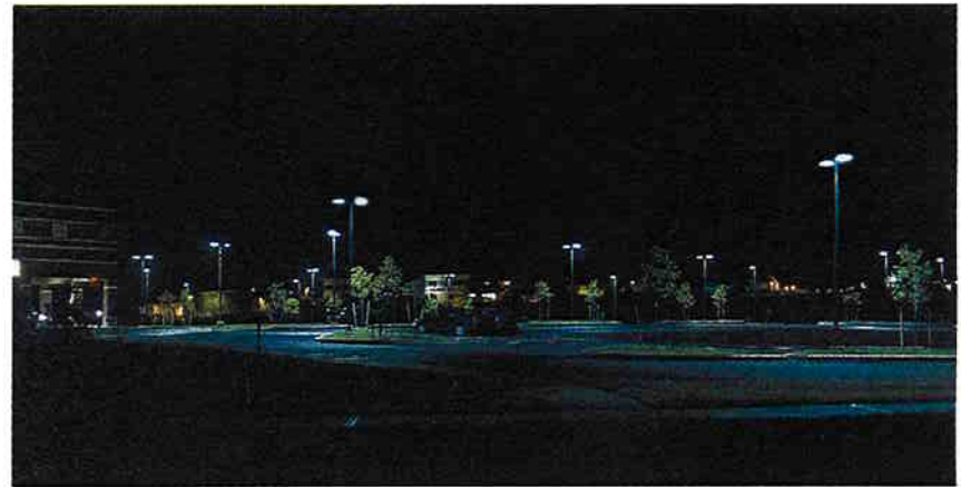
The even lighting in this parking lot facilitates visibility. Designating average to minimum light level ratios discourages severe lighting contrasts. (PHOTO: GARY CLAYTON HALL)
