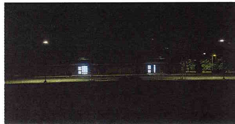
Excellent visibility for security surveillance is provided at this industrial park facility by pole-mounted cut-off fixtures and interior doorway lights. (PHOTO: GARY CLAYTON HALL)
