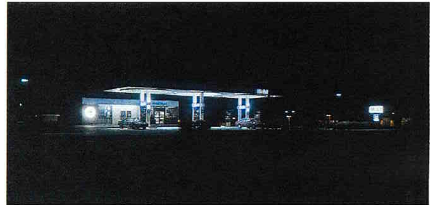
By using indirect lighting techniques, this gas station canopy provides adequate light levels without glare. (PHOTO: GARY CLAYTON HALL)
