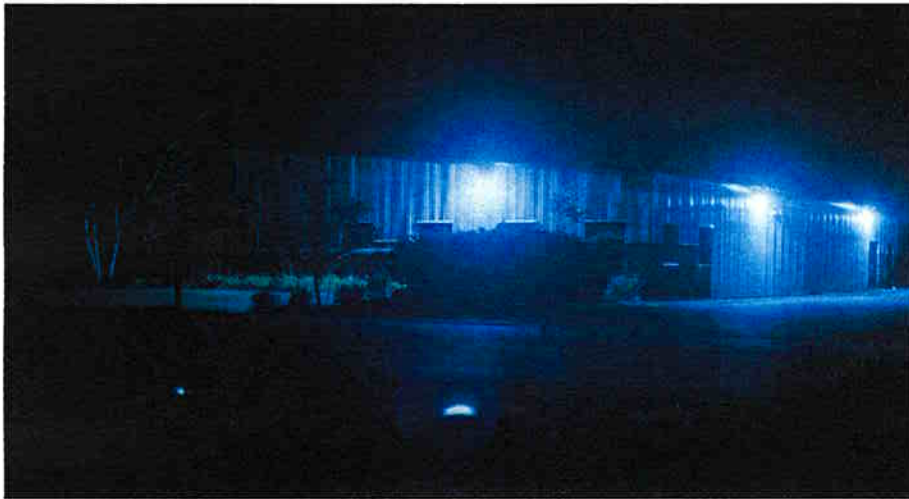
Glare from unshielded wall-mounted fixtures, installed as security lighting, makes surveillance of this industrial building difficult. (PHOTO: GARY CLAYTON HALL)
